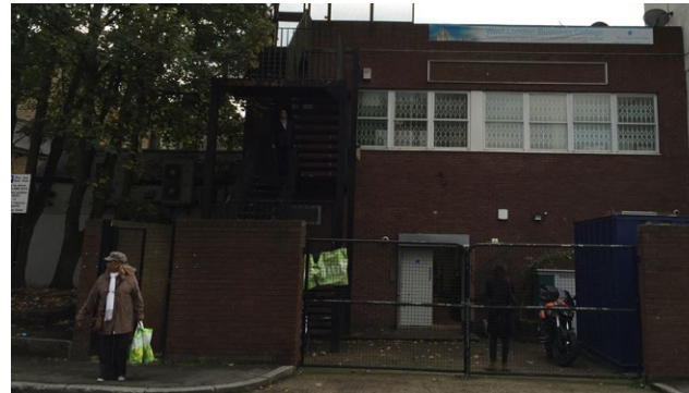
VIEW FROM THE REAR OF THE PROPERTY
