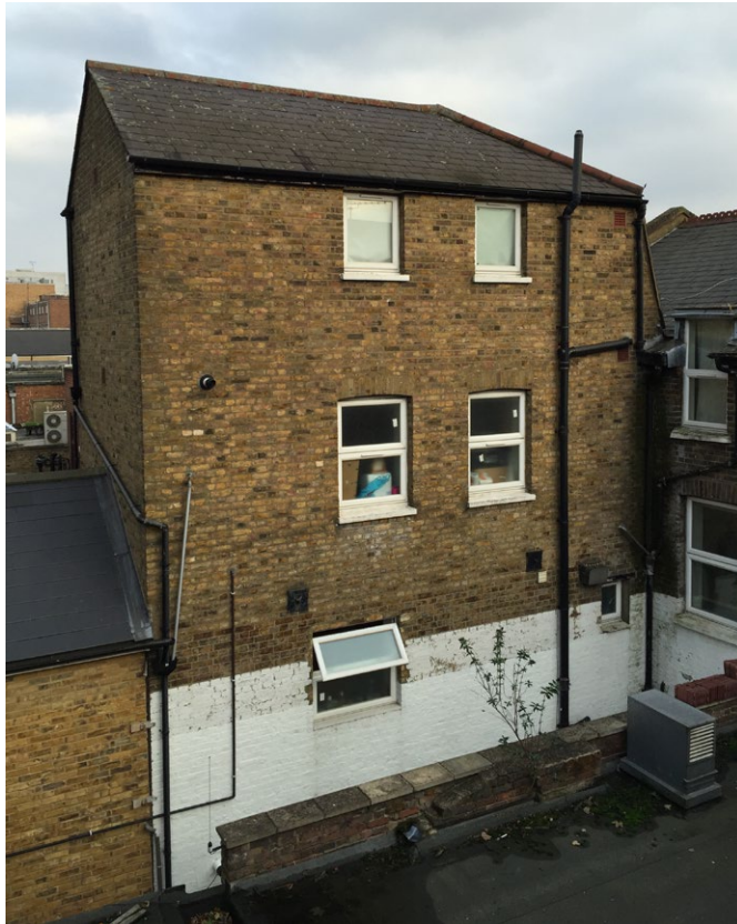
VIEW OF PROPERTY TO THE EAST FROM THE BUILDING ROOF
