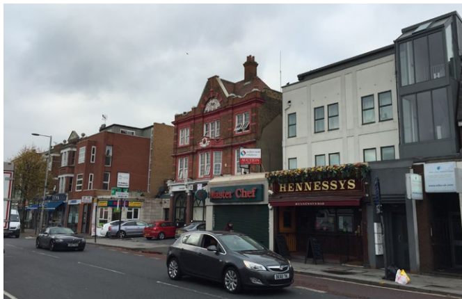
VIEW OF ADJACENT BUILDINGS
