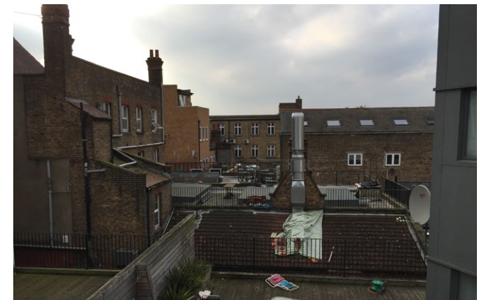
VIEW FROM THE ROOF LOOKING OVER ADJOINING TERRACES
