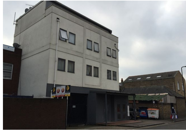
VIEW OF REAR ADJOINING BUILDING
