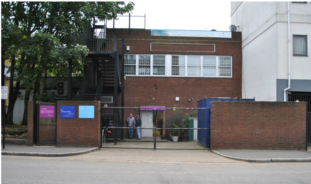
VIEW OF EXISTING BUILDING FROM SINGAPORE ROAD
